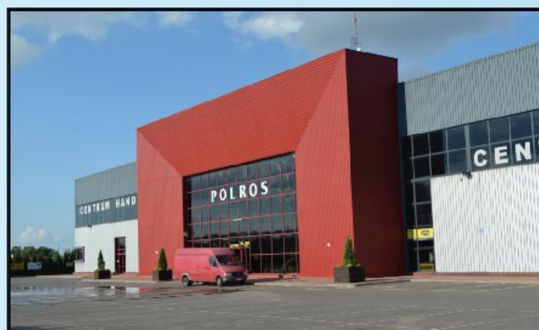
Hala Centrum Handlowego POLROS Shopping mall at the Trade Centre POLROS
